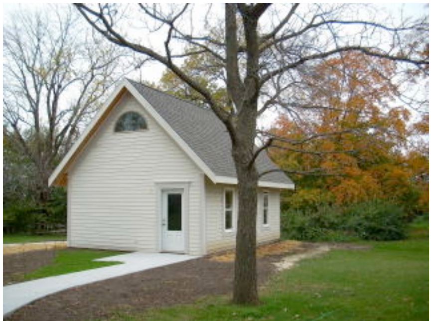
The Little Schoolhouse, built 2008 by Nick Knight and his crew using plans drawn up by Roy Knight. It is a testament to the community of memory as well as the community that still exists at Bear Creek. Its plans are a model for green technology: materials recycling and alternative energy use.
